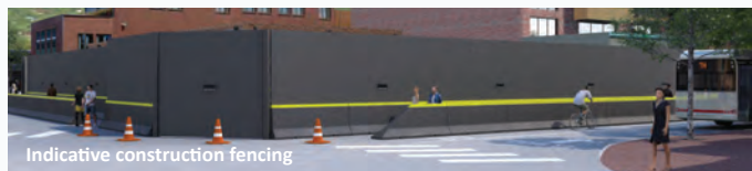
Indicative construction fencing
