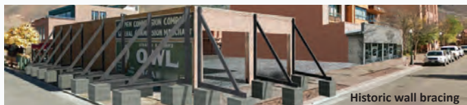
Historic wall bracing
