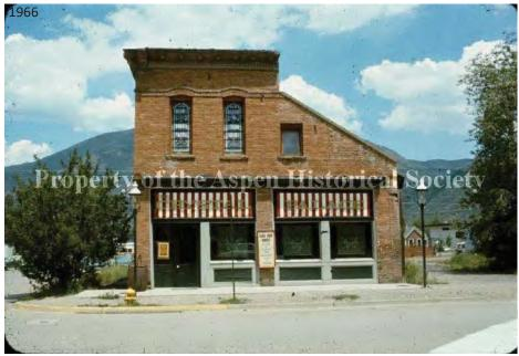
**Cornice:** A decorative cornice caps the entire building. The end brackets and corner pendant of the upper cornice matches the original photographs. As the building was expanded, the cornice was replicated to extend the length of the building on the west and south elevations. The authenticity of the dentil molding needs field verification.
