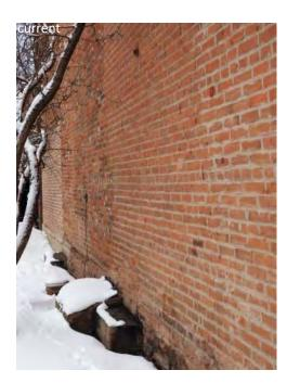
Photographs (left to right): Current photograph to show ghost image of original door location; current photograph to show concrete steps and "coal shoot".
